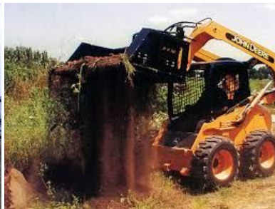
Screening Bucket at Work
